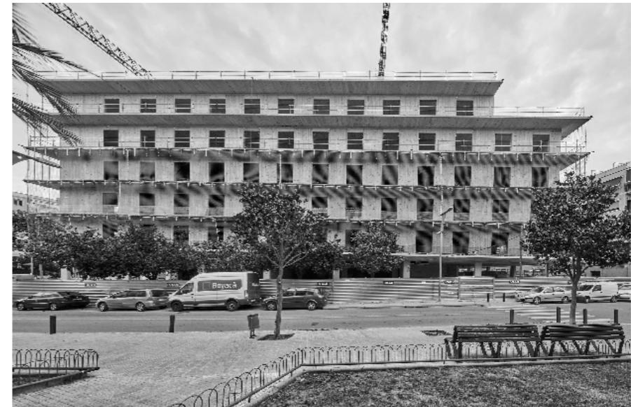
The project illustrates the potential for adopting wood as a construction system, pointing to a trend in the construction sector that has been gaining ground in European markets, due to the more sustainable nature of this modality. The facade solutions, with the combination of balconies, wooden elements and metal plates were also fundamental references for the development of this work.
