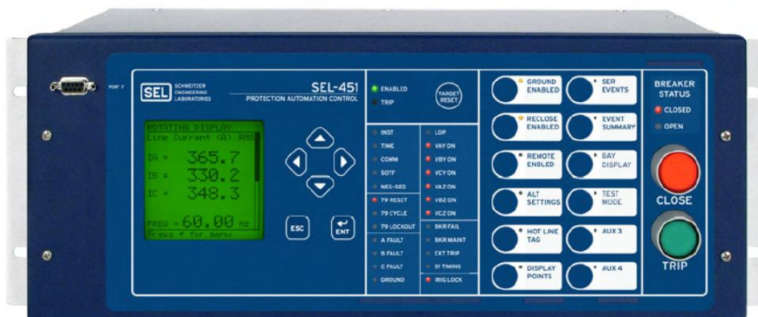
Figura 19: Vista Frontal relé digital SEL – 451
