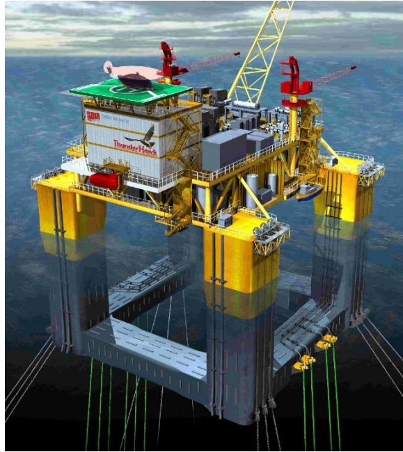
Figure 3: Example of semi-submersible platform
