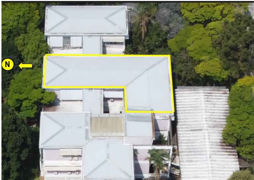
Figura 19: Bloco 4 – Central – ICMC
