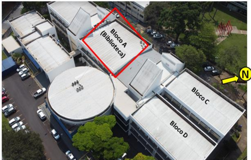
Figura 36: BLOCO A – IFSC
