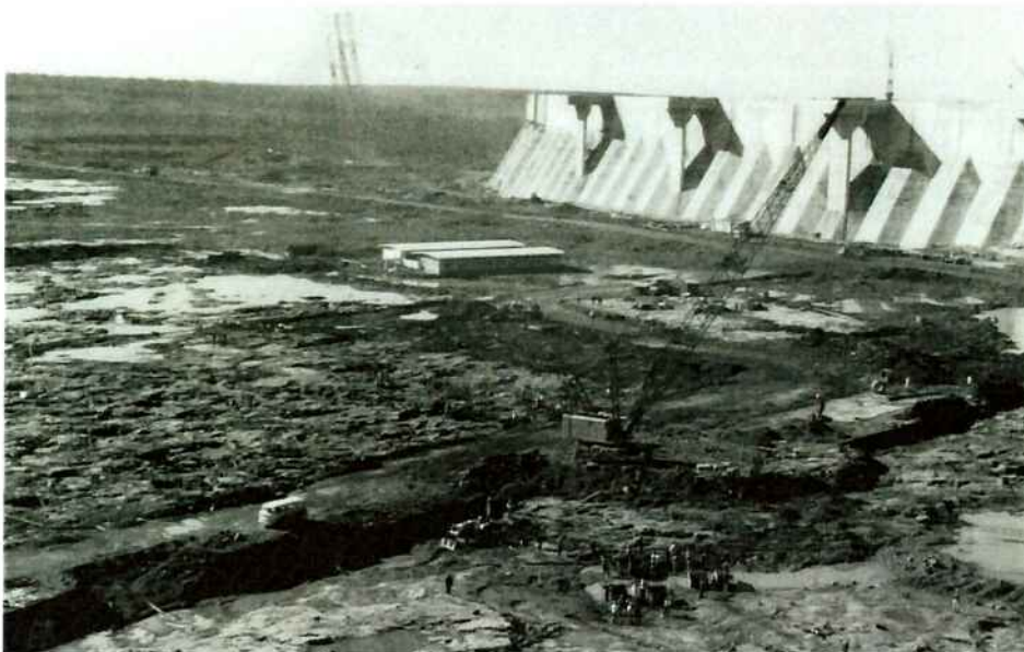
Figure 2.6 – Construction of the Itaipu Dam
