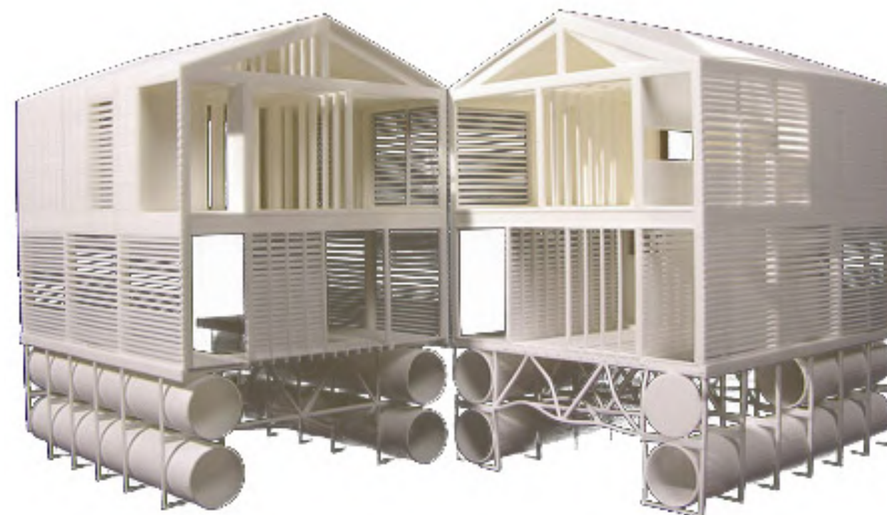
Imagem 33 - Base flutuante com barris vazios. Floating house (MOS Architects). Fonte: < https://www.archdaily.com/10842/floating-house-mos >. Acesso em: 30/02021
