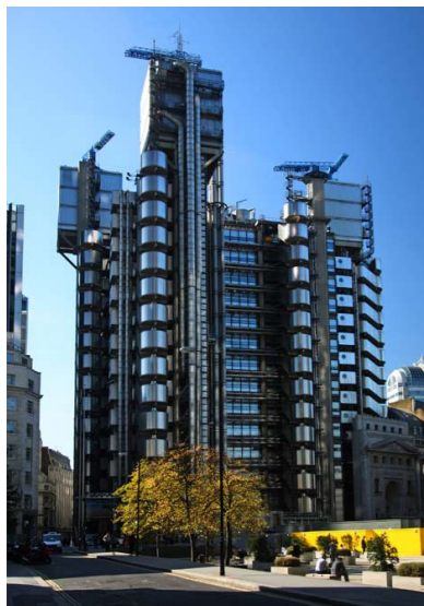
Figura 6: Edifício Lloyds Bank. Fonte: https://www.dezeen.com/2013/08/04/movie-richard-rogers-lloyds-building-high-tech-architecture/
