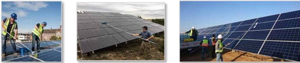
Figure 8 - Visual examples of the manual cleaning process
