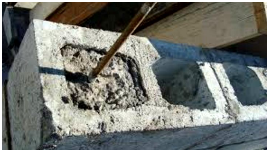
Figura 19 - Bloco Grauteado e Armado (fonte: http://4.bp.blogspot.com/-x131GKAdQXE/UvQpBe4xt6I/AAAAAAAAAD50/8QEzDh9iOV0/s1600/preview_html_5f34c62f.jpg )
