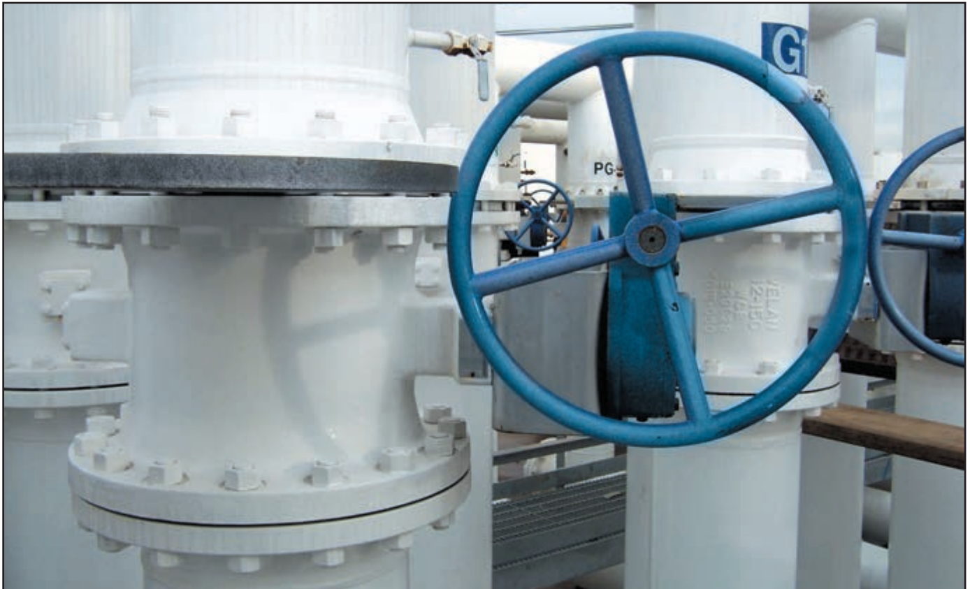
Torqseal® triple-offset valves, NPS 12 (DN 300) in a tank farm manifold.
