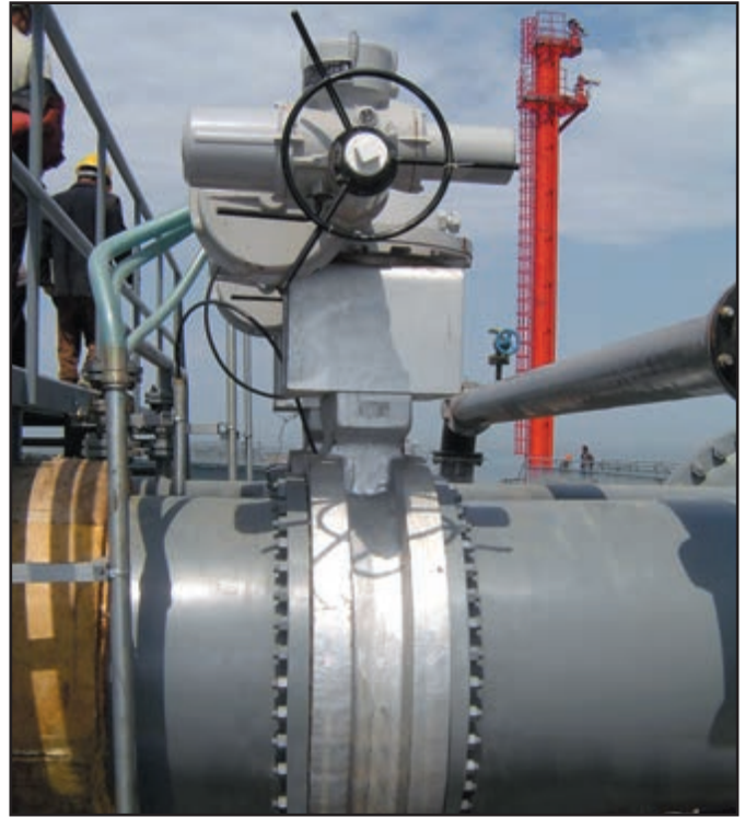
Motor operated NPS 36 (DN 900) Torqseal® in crude oil.
