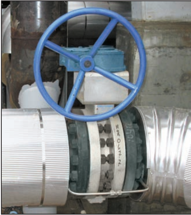
NPS 12 (DN 300) Torqseal® triple-offset valve for steam isolation.
