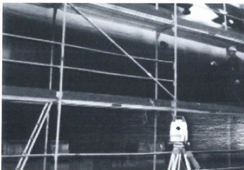
Picture 6: Single operator 3D-roundness check using a total station (3D measurement)
