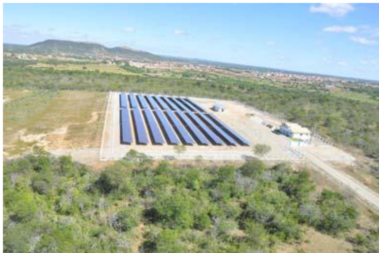
Figura 3 - Usina Solar Tauá - Tauá/CE [14]
